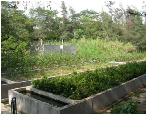
Constructed mangrove wetland treatment belt in Shenzhen
