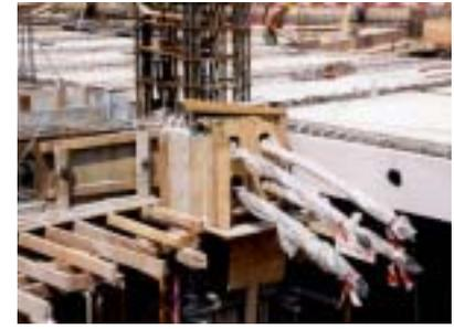
Figure 21 – Deck using precast beams and semi-slabs strengthened by post-tensioning arrangement
