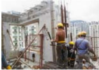
Figure 17 – Lost-form is used for external wall (for walls without window opening)
