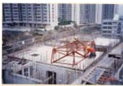
Figure 2 – Semi-precast slab system used in Harmony project
