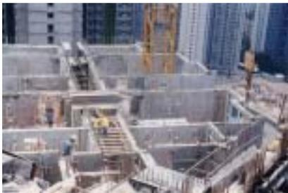
Figure 22 – Access problem may be created during installation of the precast units
