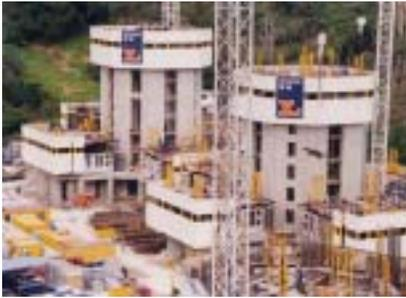
Figure 16 – HKHA Concord project using Jump-form for core wall and precast façade for external walls
