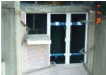
Figure 5 – In-situ grouting to joints between façade and external walls
