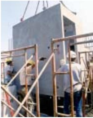
Figure 19 – Precast toilet cubicle for a public housing project
