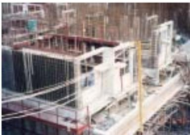
Figure 7 – Casting the façade together with the structural wall
