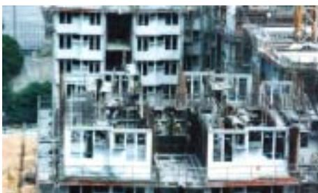
Figure 1 – Use of precast façade in HKHA’s project under Harmony Design
