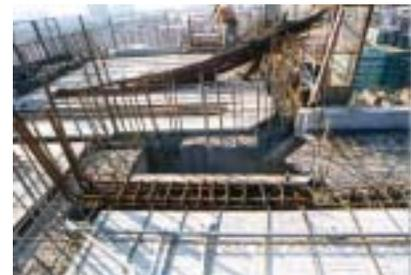
Figure 24 – Several pieces of precast elements joining together requires accurate dimensional coordination
