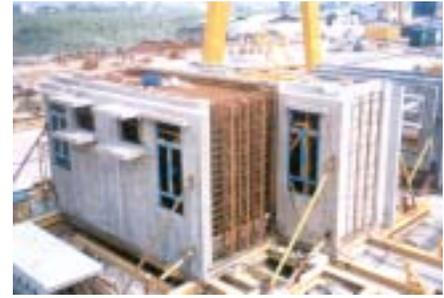
Figure 18 – Modulated precast unit for an experimental project developed by Gammon Construction Ltd.
