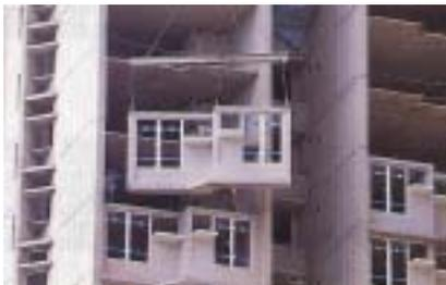
Figure 4 – Fit-in façade for the first generation of housing projects
