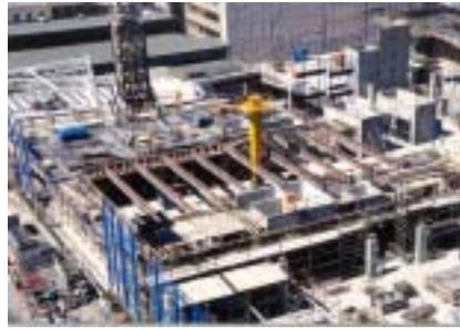
Figure 20 – A hybrid construction system using precast panels for the core and floor supported with steel beams
